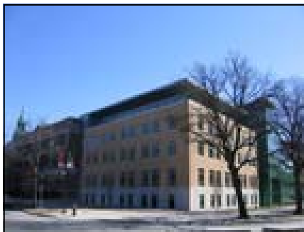
Corner view of the new Library building
