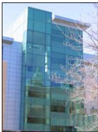
Modern, glass tower welcomes users to the new Library
